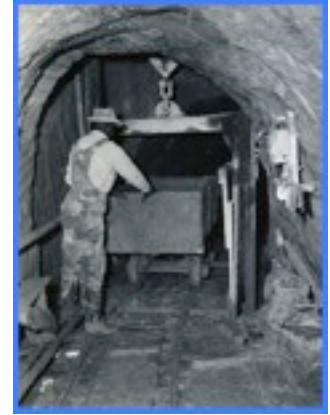
Edisto River water supply tunnel construction, 1928
